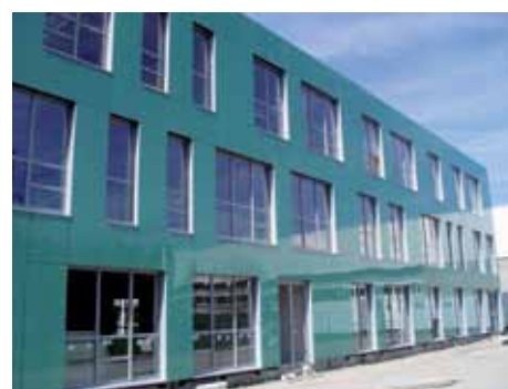
Papendal Arnhem Architect: Hooper Architects
